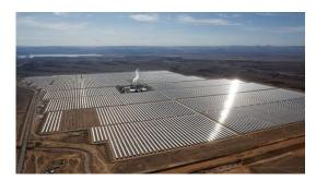
**Noor 1** Ouarzazate Solar Power Station (OSPS) – Phase 1, also referred to as **Noor I CSP**, has an installed capacity of 160MW. It was connected to the Moroccan power grid in February 2016. It covers 1,112 acres and delivers 370 GWh per year. The plant is a parabolic trough type with a molten salt storage for 3 hours of low-light producing capacity. The cost of the project when it began operations was \$3.9 billion. It uses half a million mirrors.
