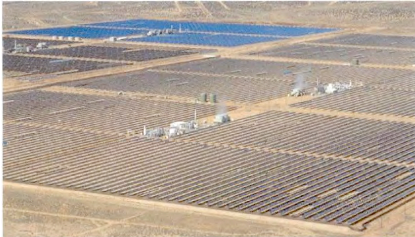
Figure 6: Solar Trough Plant at Kramer Junction
