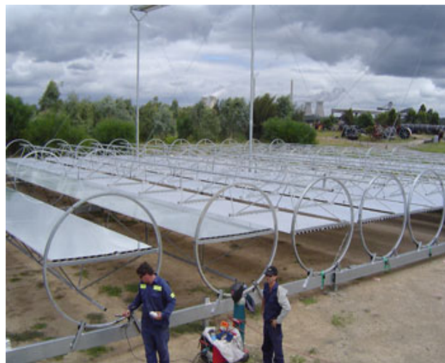
At the Liddell coal fired power plant, concentrating solar power preheats water to reduce coal usage
