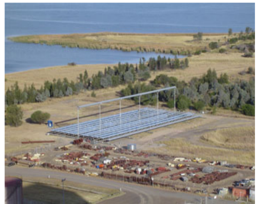
Aerial view of the Liddell solar field
