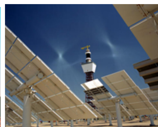
Concentrating solar power towers
