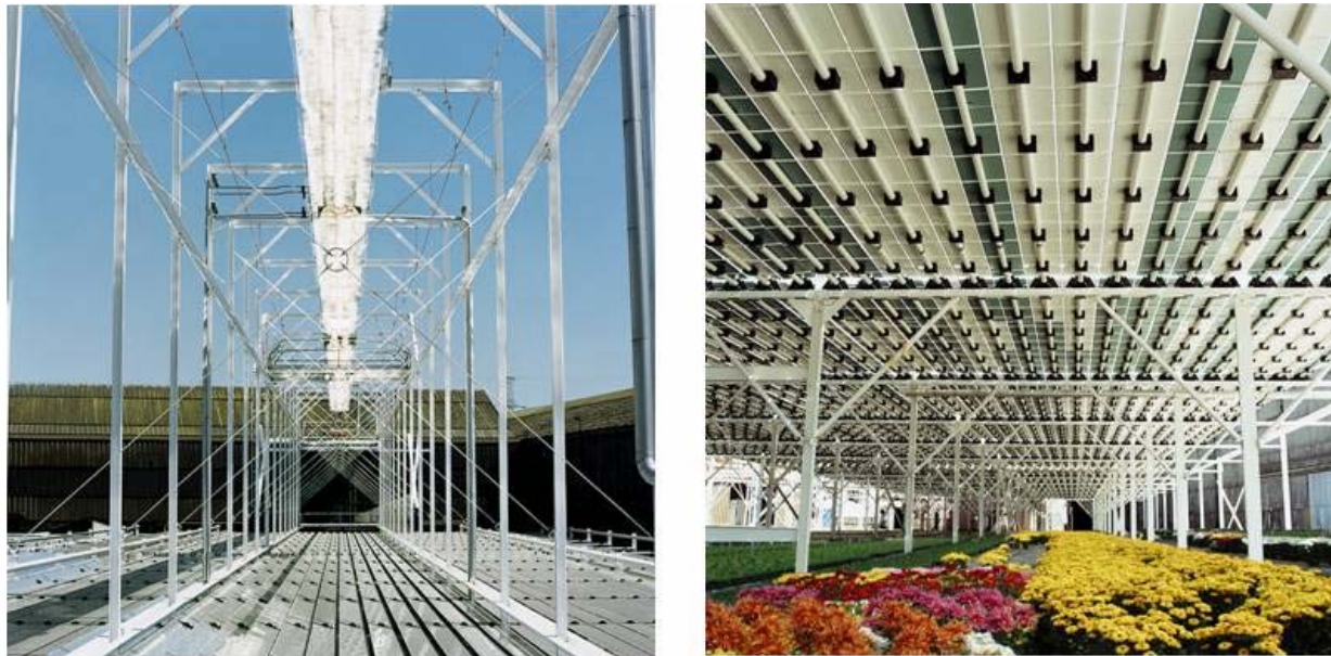
Figure 2-41: Photo of the top of a Linear Fresnel Concentrating Solar Collector and artist view of a greenhouse installed underneath to protect the plants from excessive irradiance and evaporation. This could be a concept for multi-purpose plants for power, water and horticulture. Other local uses include shade for parking and the production of steam for cooling and process heat. Source: Solarmundo, DLR)
