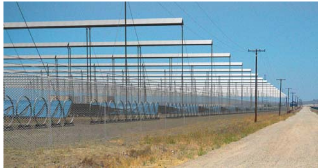
Figure 1. Visualization of the proposed 177 MW plant at the Carrizo Plain, California. Tracking linear reflectors focus solar energy on elevated boiler tubes to produce steam.
