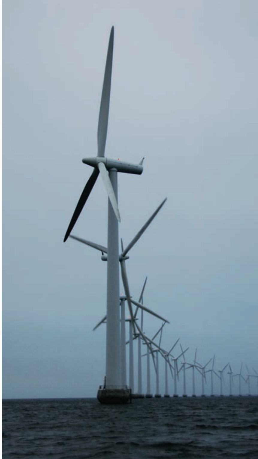
The 20-turbine Middelgrunden wind farm, installed in 2000, produces 90 megawatt-hours of electricity a year. PHOTO BY BENJAMIN K SOVACOOOL
