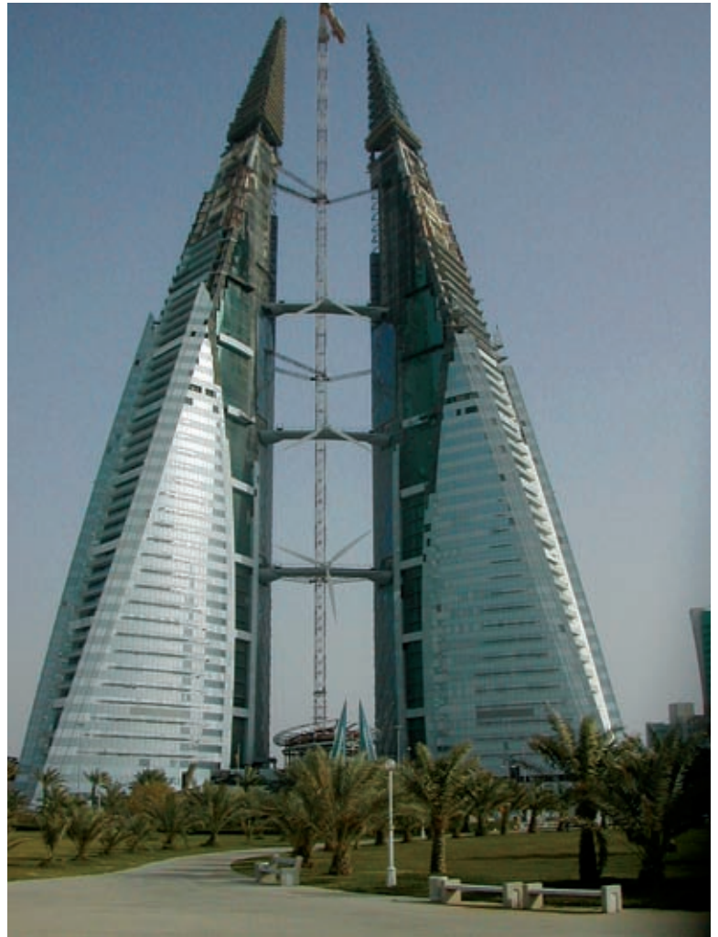
The new Bahrain World Trade Center sports three wind turbines made by Norwin and engineered by Ramboll, both of Denmark, that will generate up to 15 percent of the building's electricity. PHOTO COURTESY OF RAMBOLL
