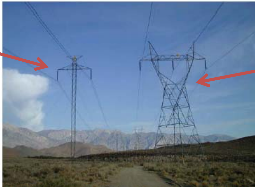
Figure 1-B. Left powerline: The Pacific Direct Current Intertie (PDCI), near Bishop, CA. HVDC, 3,000 MW, +/- 500 kv bipole, 846 miles from Celilo, at The Dalles Dam, OR to Sylmar (NW Los Angeles, CA). Commissioned in 1970 as 1,500 MW line. The right powerline is conventional high voltage AC.
