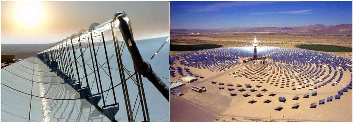
Figure 20: Examples of Concentrated Solar Powers: Parabolic Trough System and Solar Tower System
